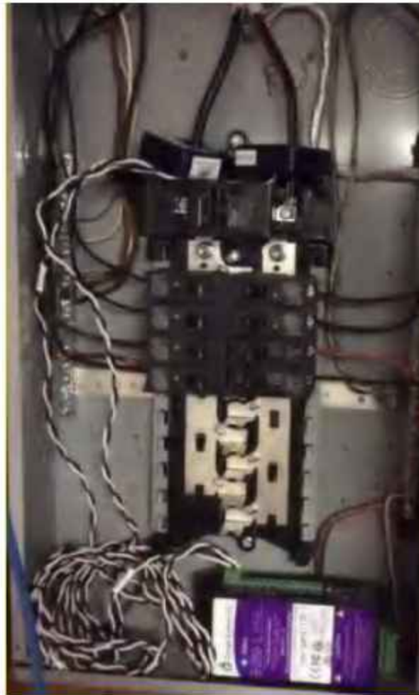
Figure 2-9. Example eGauge 3010 Installation
